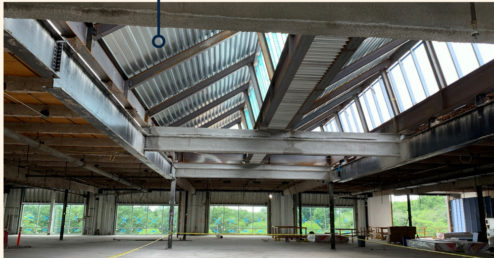
During Construction April 2022
