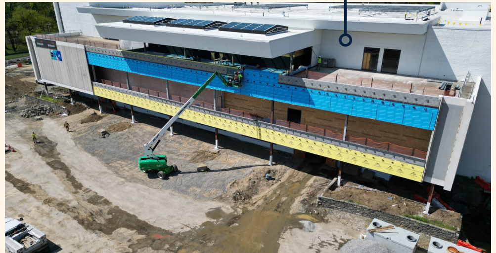
During Construction April 2023
